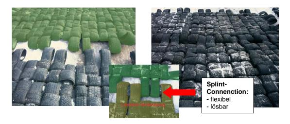
Mat / crosswise netting, precast modules, connectable to any faces, can be taken off and are reusable more than hundreds of times.
